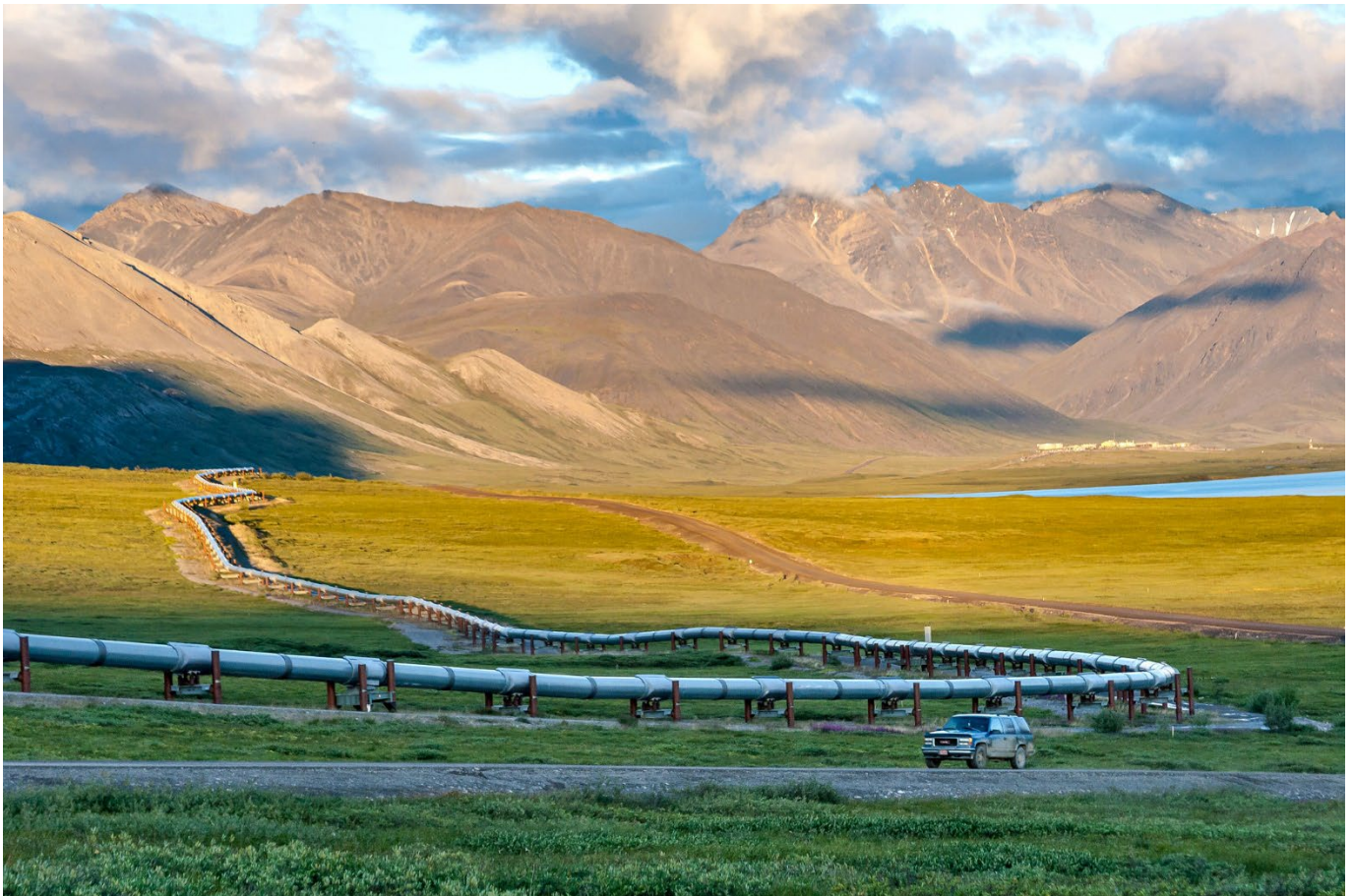
Image 1. Trans-Alaska Pipeline Near Galbraith Lake on the Dalton Highway
