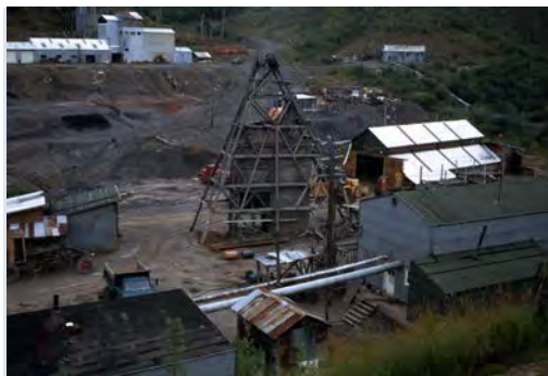
The Pre-1955 Main Processing Area, showing headworks and support buildings. The post-1955 mill is in the background.
