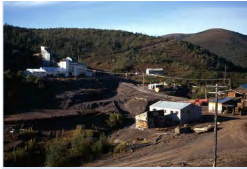
The Main Processing Area in 1969, showing the flotation mill added to the post-1955 mill building, and the settling ponds.
