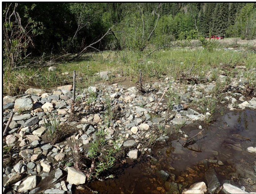
Figure 49. Several live stakes starting to grow along a streambank.
