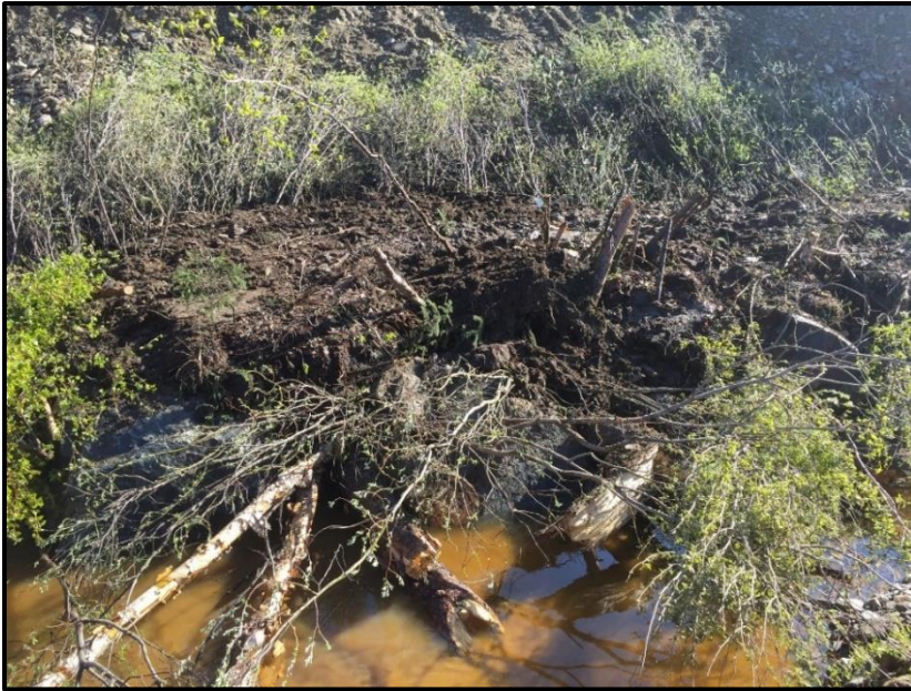
Figure 39. Boulder and log toe protection with transplants placed on top. Live cuttings are included with brush. The large wood and brush cuttings were placed between the boulders.
