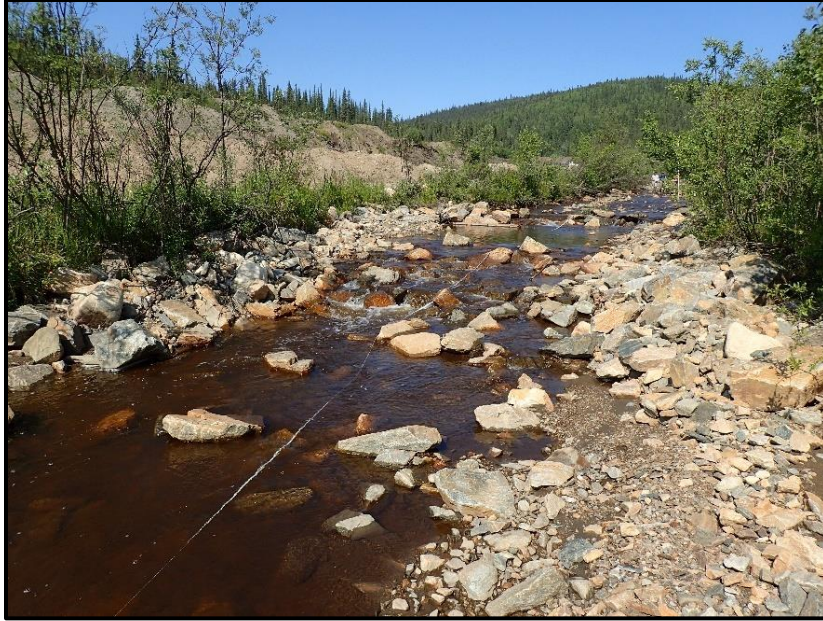
Figure 66. Riffle incision at the downstream end of a constructed riffle.
