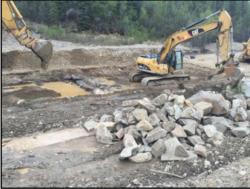
Figure 53. Track hoe with hydraulic thumb (right) installing a constructed riffle.
