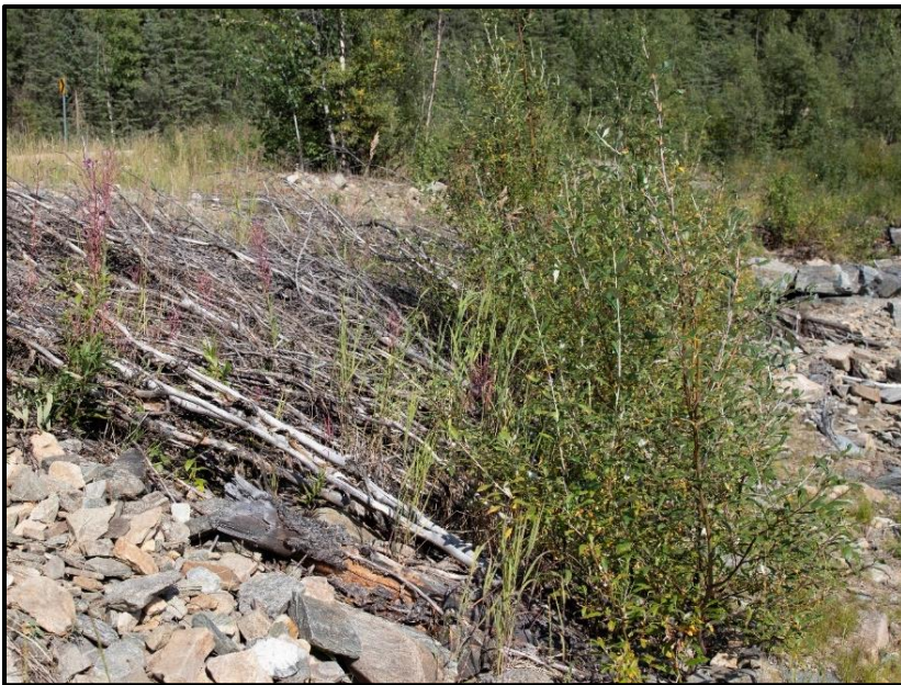
Figure 47. Another brush mattress on the same project site as previous figure. Note the willow growth from the base of the structure. This growth is supported by the contact of the mattress with the water table.
