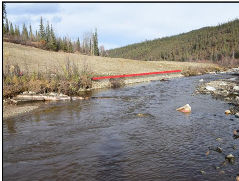
Figure 61. Erosion and loss of streambank transplants. Red line shows bank length that has eroded.
