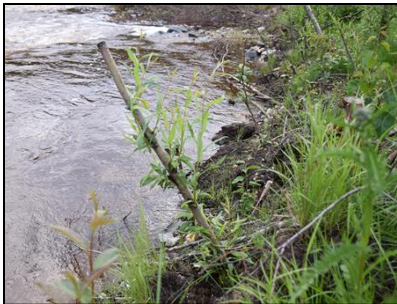
Figure 48. Live stake sprouting shortly after installation.
