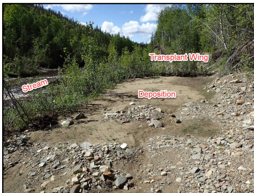
Figure 50. Transplant wings with sediment deposition upstream.
