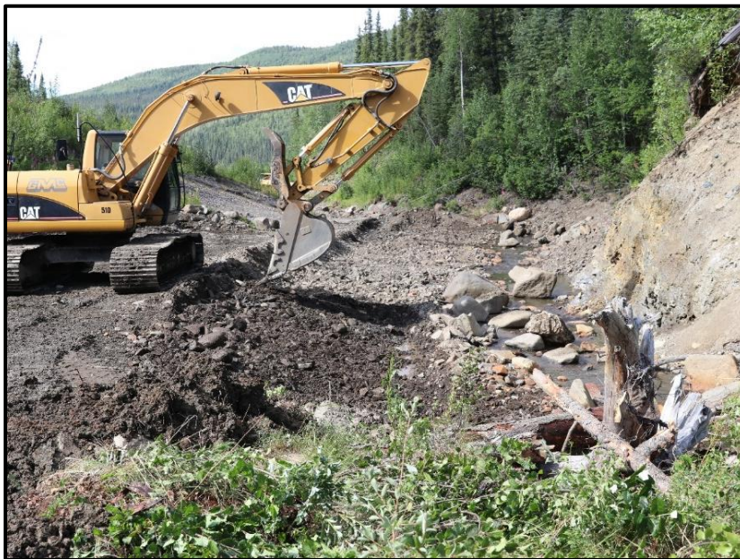
Figure 42. Preparing the site for transplants by excavating a shallow trench beside the stream channel. Transplants are placed in the trench.
