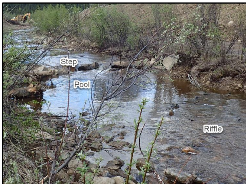
Figure 37. Constructed step-pool structure.
