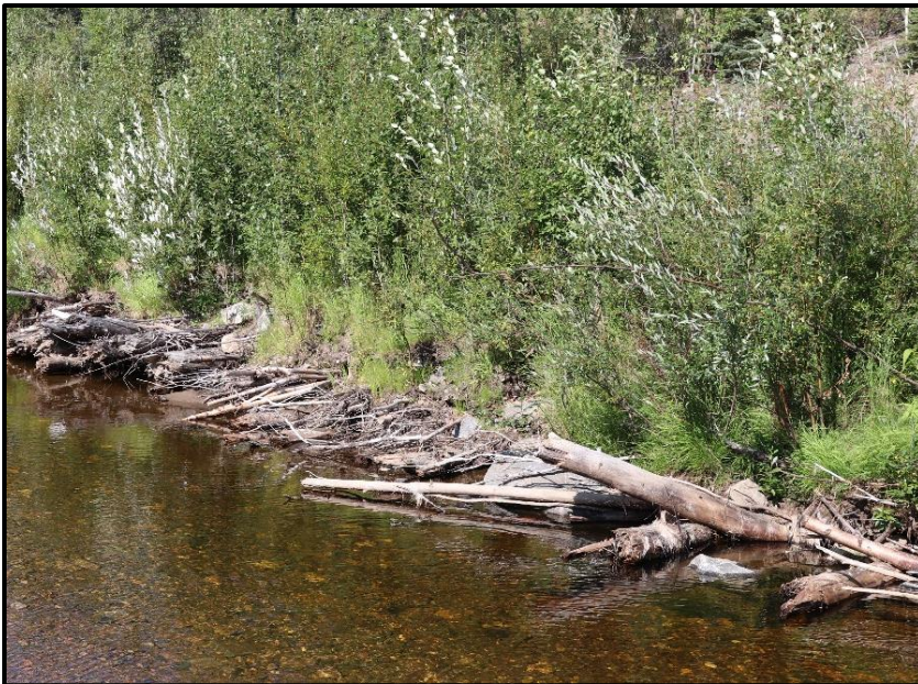
Figure 40. Same bank as Figure 39 showing the boulder/log toe protection and a bankfull bench with transplants three years after construction.
