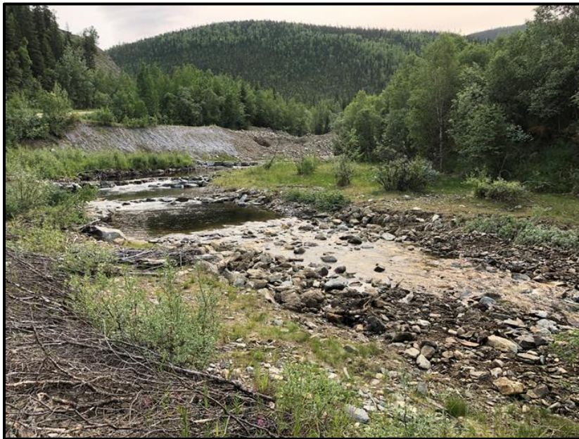
Figure 36. Riffle (from previous figure) after construction has been completed.
