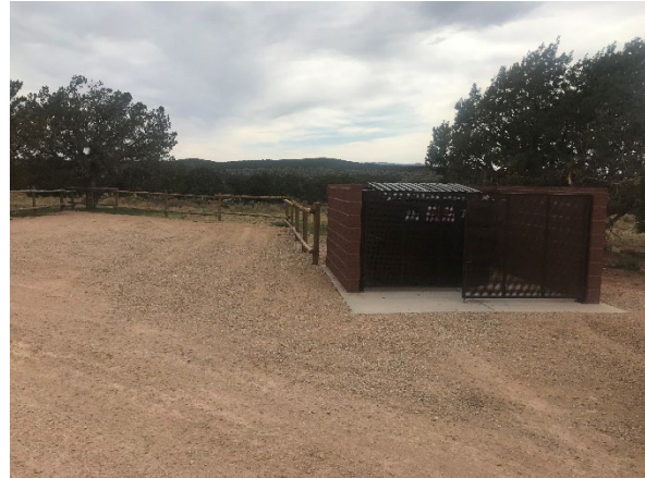
Trash Receptacle at Pyramid Ridge Campground
