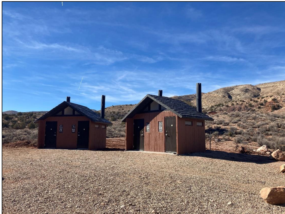
Photo 3: Newly installed vault toilets at the Wire Pass Trailhead.
