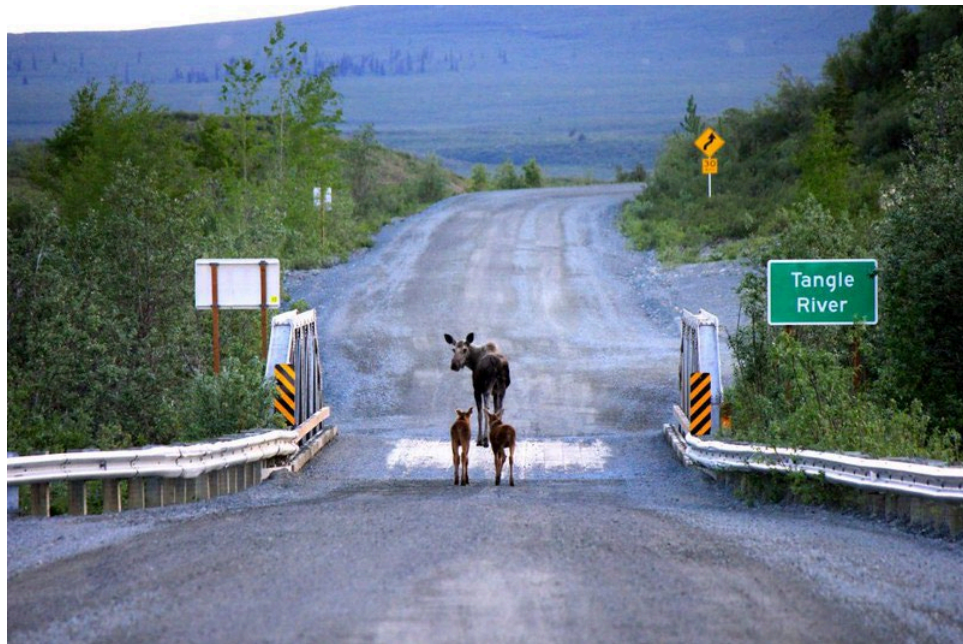
Tangle River Bridge adjacent to Campground Entrance Road
