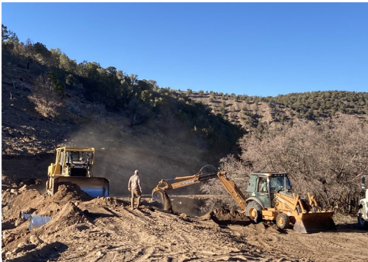
Breaking Ground At Sauls Meadow Campground
