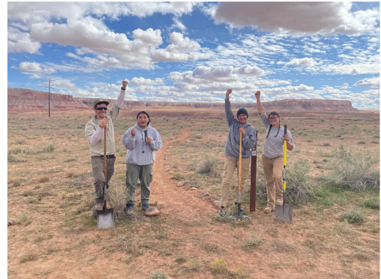
Canyon Country Youth Corps and BLM building trail
