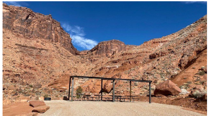
Big Bend C Group Site Remodel
