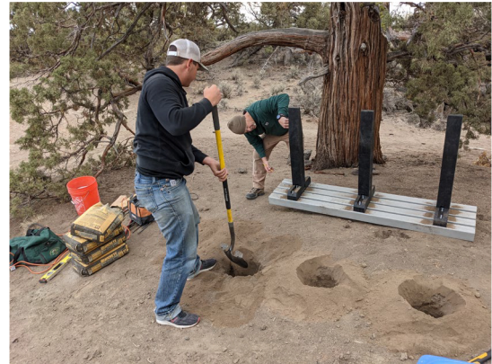
Recreation staff installing benches.
