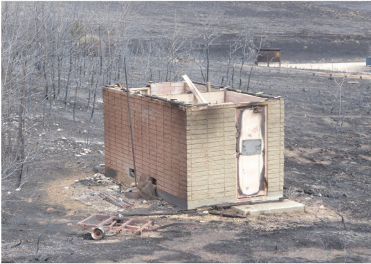
Vault removal from a burned vault toilet
