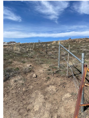
Fence repair supports the multiple-use mission.
