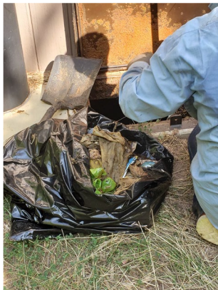
Contractors remove trash from a toilet vault
