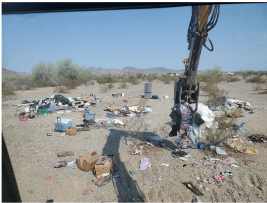
Heavy Equipment Cleanup
