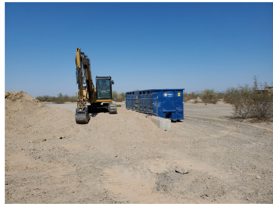
Heavy Equipment Finalizing Access Ramp
