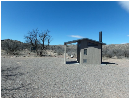
New vault toilets at Fourmile Canyon Campground
