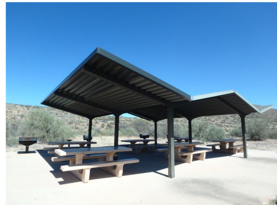
Flying "W" Group Site repaired roof
