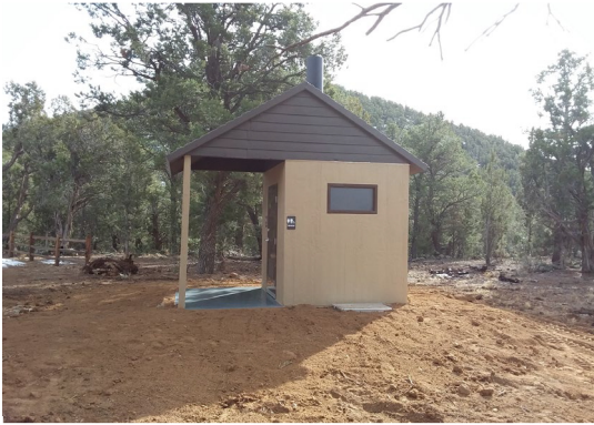
New Vault Toilets
