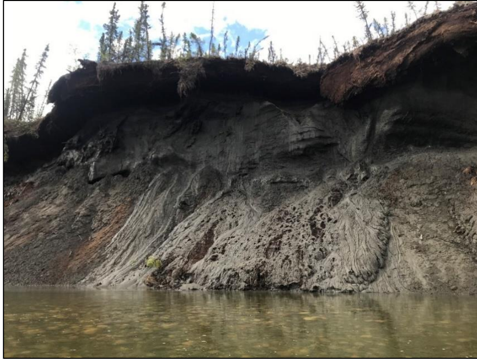
Figure 8. Streamside photograph showing unstable embankment, melting permafrost area, lower Birch Creek Wild and Scenic River. BLM photo by Teri Balsler.
