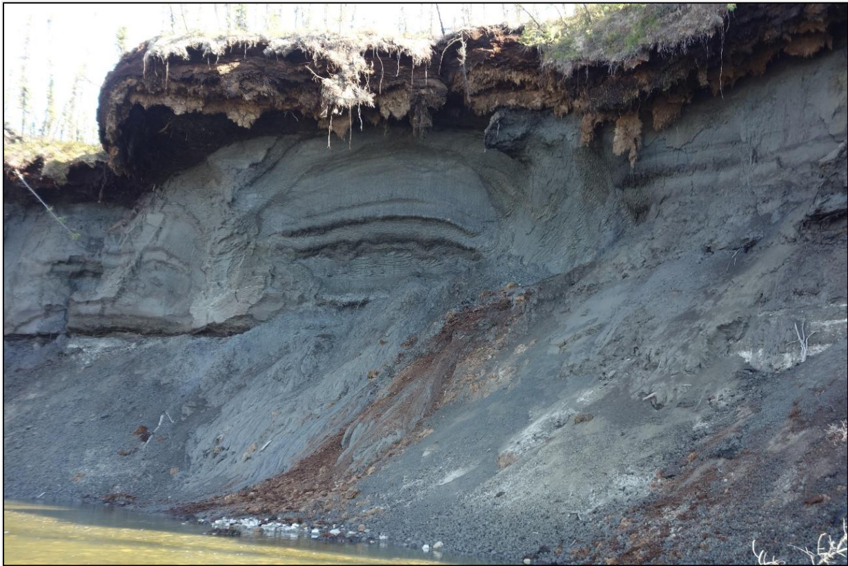
Figure 11. Streamside photograph showing unstable embankment, melting permafrost area, lower Birch Creek Wild and Scenic River, June 2020. BLM photo by Robin Mills, BLM
