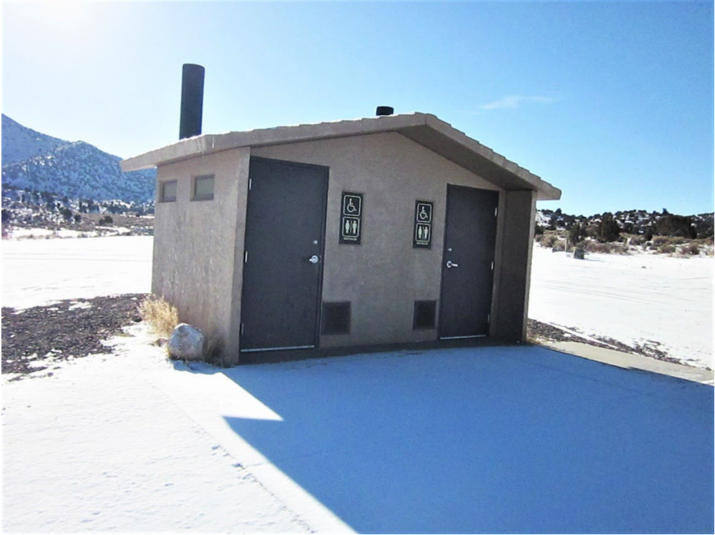
Photo 5: Close-up view of double-vault restroom facility
