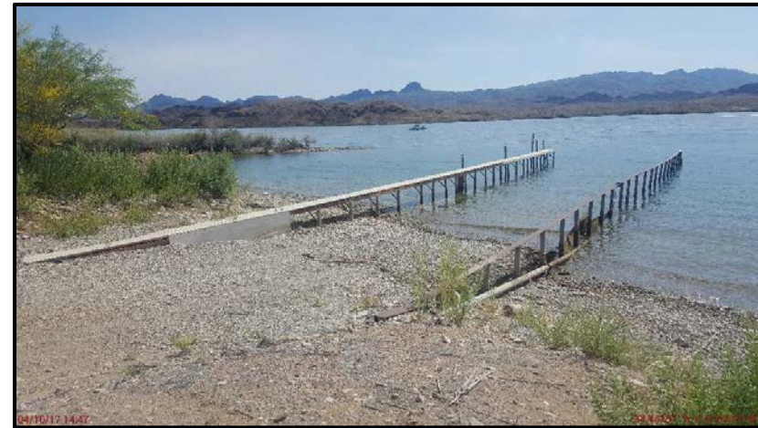
Existing ramp and dock.
