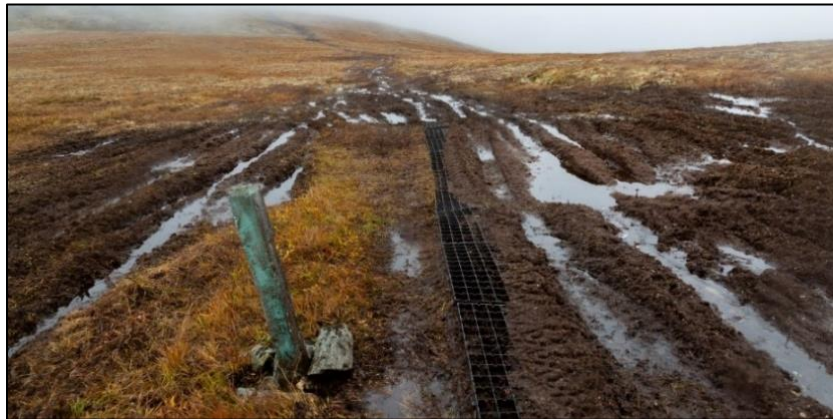
A section of trail-hardening geoblock on the Pinnell Mountain NRT covered in mud after off-highway vehicles severely impacted over a mile of the non-motorized hiking trail near Eagle Summit.
