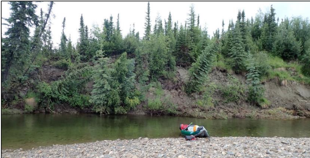
Large embankment slump/debris slide on Birch Creek WSR near the confluence of Harrington Fork, July 13, 2020. Inflatable canoe in center foreground for scale.
