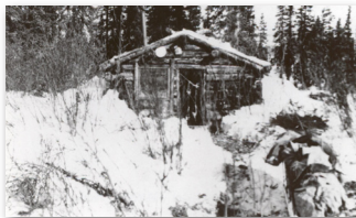
4-Mile Trapper Cabin
