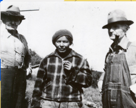
Horace Wickersham, Anne, and L.S. Wickersham at Valdez Creek, Alaska.
