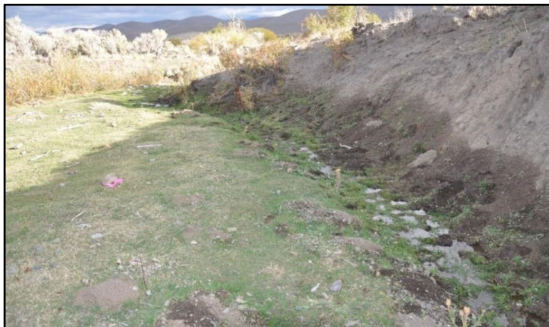
Figure 26. Upper part of the Ferris Creek DMA looking downstream.
