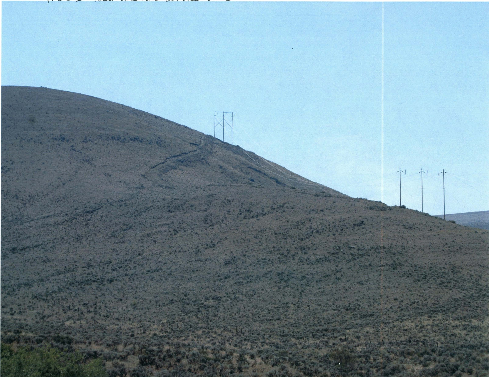
Frame 1: Power line and Service Road
