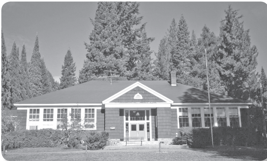
Pineburst School in the wildland-urban interface.
